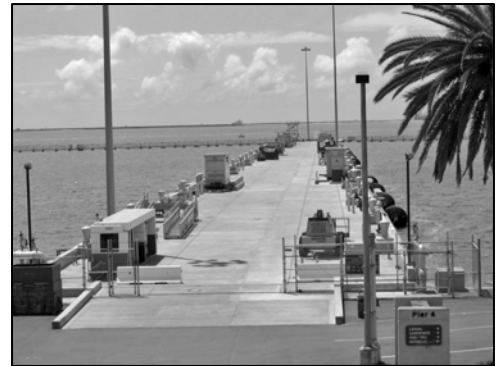
Pier 4 After Repair
